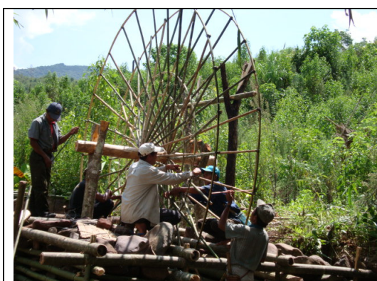
Mr Song building a water wheel with other villagers as part of the on the job training
