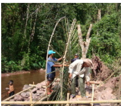
Building of gabion dam and water wheel
